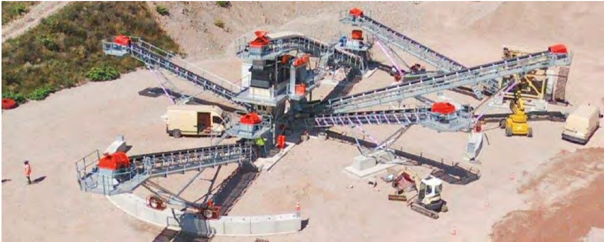
Figure 15: The new permanent crushing and screening installation. Sablières J. LEONHART.
