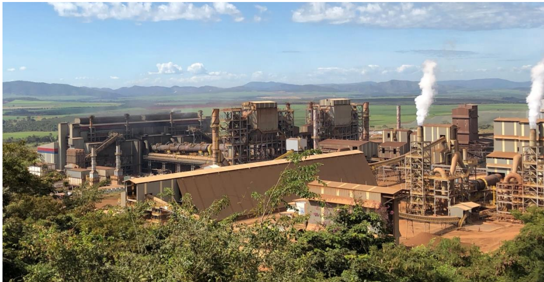
Figure 4: 29 th May - Visit to the industrial plant at the Barro Alto Complex, operated by Anglo American.
