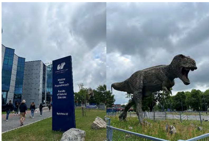
Fig3: External view of the Institute of Earth Sciences in the Faculty of Natural Sciences.
